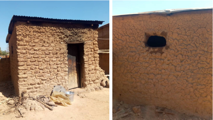
A mud block house in Ziasso village, with new ventilation window in kitchen
